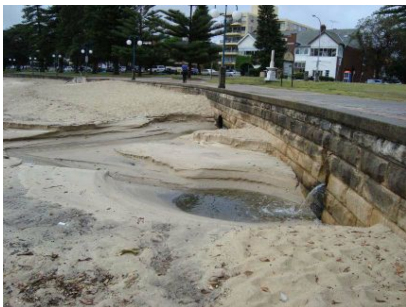
Figure 10.4.2a – Scour from stormwater outlets, Manly Cove East Beach.
