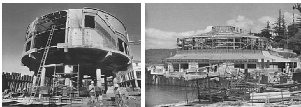
Figure 5.16.2k & 5.16.2l - Demolition of Marineland, 1987 and construction of Oceanworld, 1988
