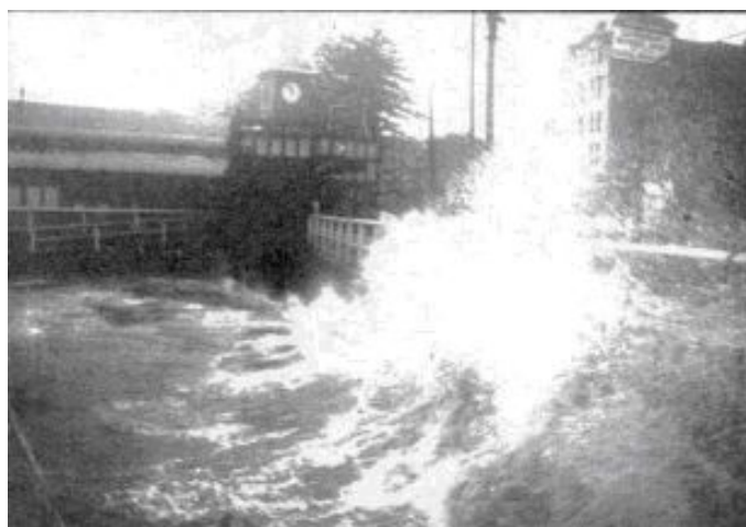
Figure 6.4 – Wave overtopping of Manly Cove east seawall during 1974 storms
