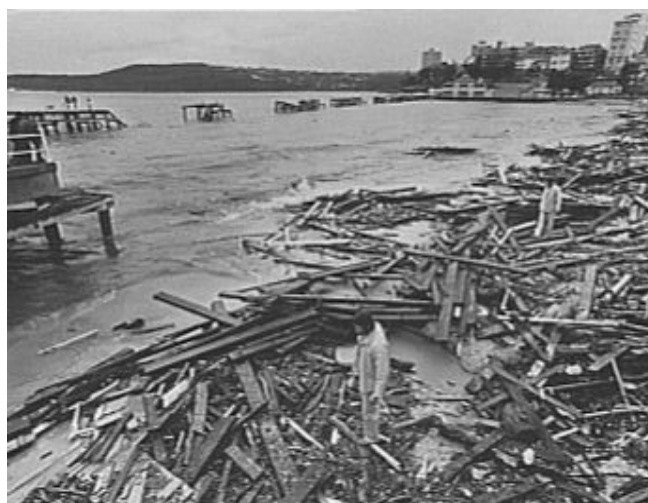
Figure 5.15.1b – Destruction resulting from 1974 storm activity
